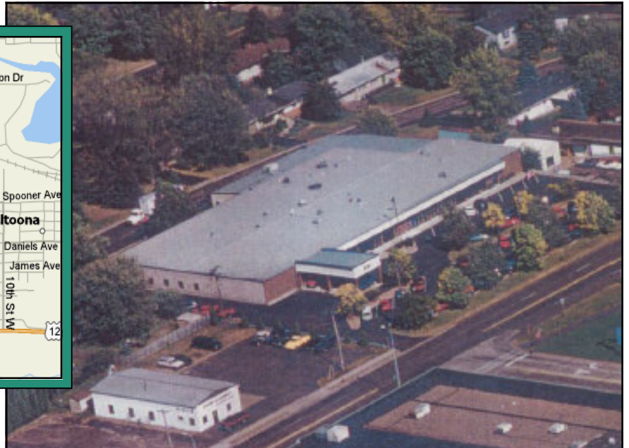
Aerial View of Building
